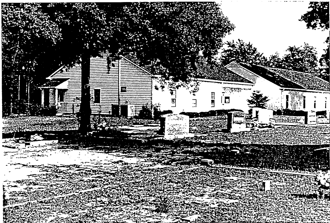
NEW EDUCATIONAL BUILDING 1984 (NORTH SIDE)
