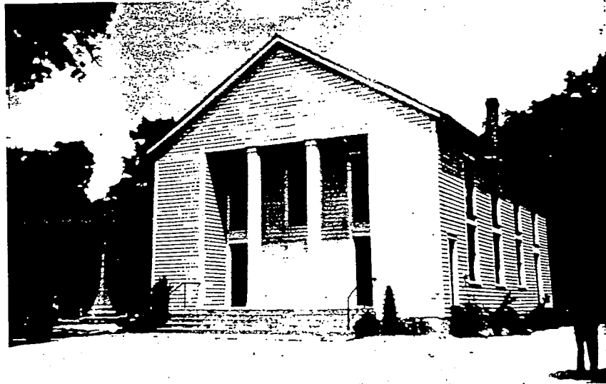
SANDY LEVEL CHURCH SANCTUARY BUILT 1856
